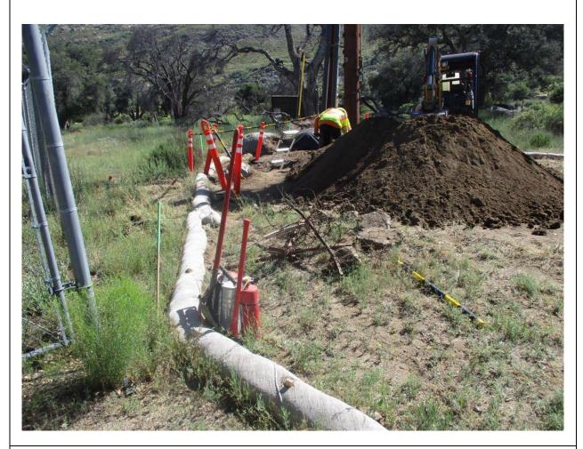
**Photo 3:** During excavation work to install intercepts at P161903 (C 449), perimeter fiber rolls were observed functional in accordance with the ECP and SWPPP. A complete set of fire tools was staged on site (5-gallon backpack pump, round point shovel, Pulaski, and 2A10BC fire extinguisher) in accordance with the CFPPP (MM FF-1).
