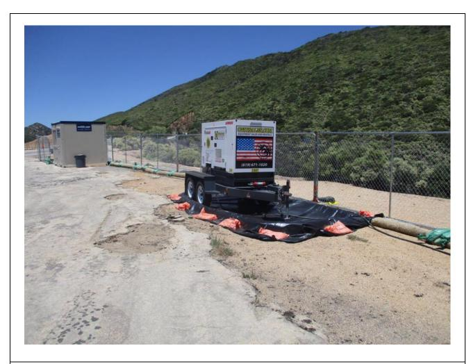
**Photo 6:** Visqueen was observed staged beneath a stationary generator at a C 440 staging yard for drip and spill protection in accordance with the SRNP and MM PHS-2.
