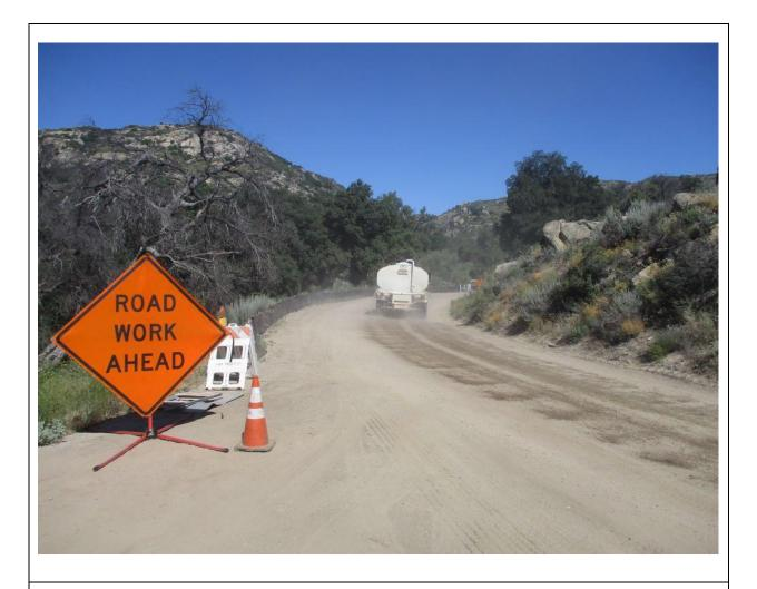
**Photo 5:** A water truck was observed being used to control fugitive dust emissions along Corral Canyon Truck Trail in accordance with APM AIR-02 and APM AIR-05. Traffic control signage was also observed along the road in accordance with the Traffic Control Plan.
