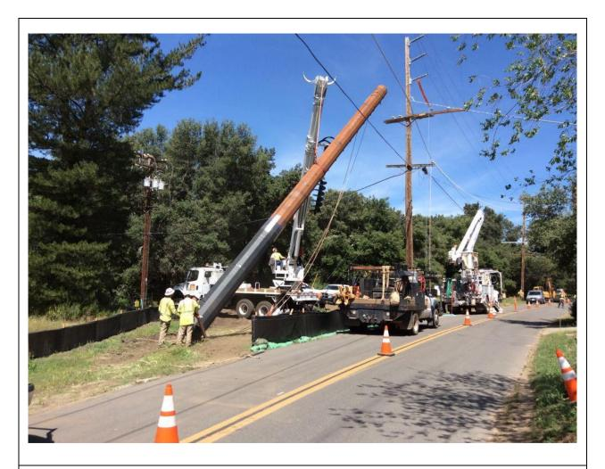
**Photo 2:** A construction crew was observed setting the pole base at Pole Z172804 (TL 629A). Cones, signage, and traffic flaggers were used to maintain a safe travel corridor for motorists in accordance with the Traffic Control Plan and APM TRANS-02. Arroyo toad exclusion fencing was observed in good condition with gravel bags in accordance with arroyo toad avoidance and minimization measures (APM BIO-03).
