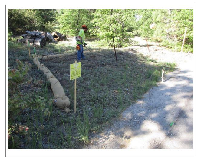
**Photo 4:** While a construction crew was performing vegetation clearing at a vault along C 440, ESA signs were posted to notify crews that cultural resource monitoring was required at this location per Appendix A of the HPMP. Staking and flagging clearly delineated approved workspace in accordance with MM BIO-1.
